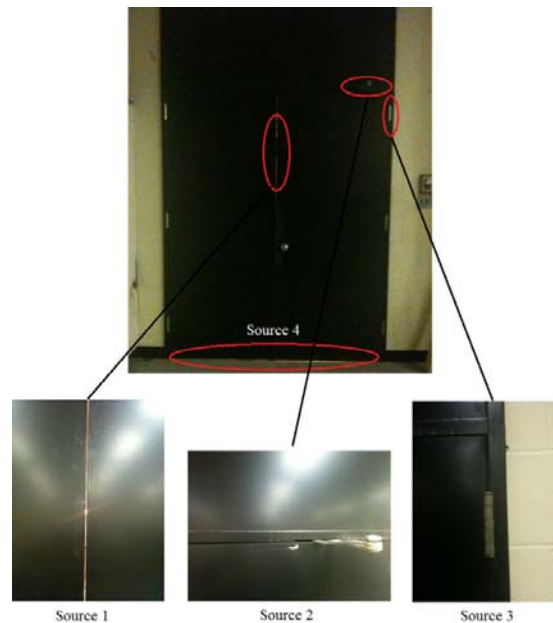
Fig 5. Schematic of the door with major air leakage spots indicated. A mechanically-driven pressure difference existed across the door under normal building operation.
