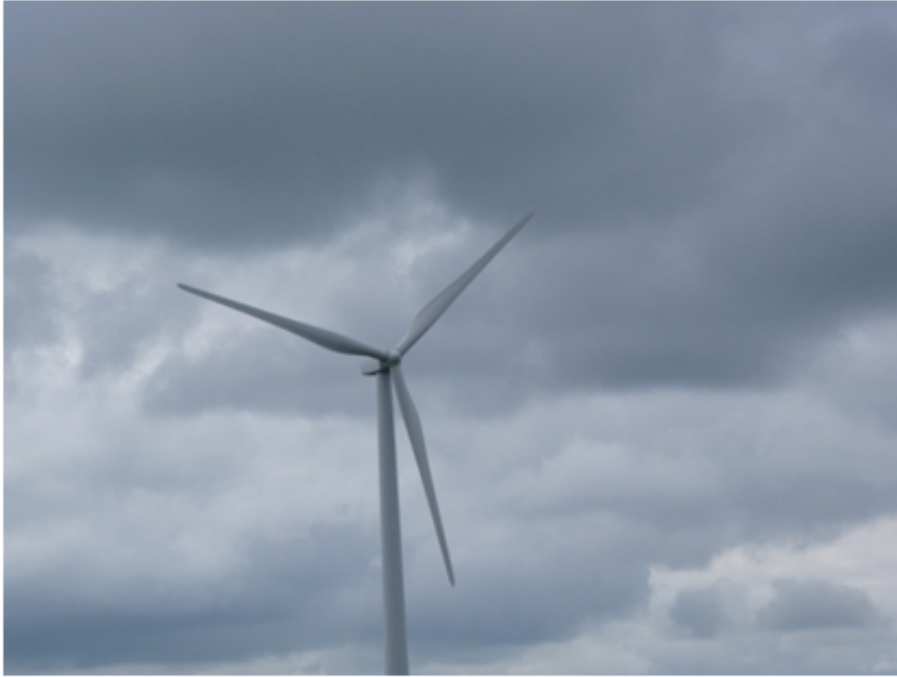
Figure 4: The GE 1.5 MW wind turbine located at the Invenergy wind farm in Grand Ridge, Illinois.
