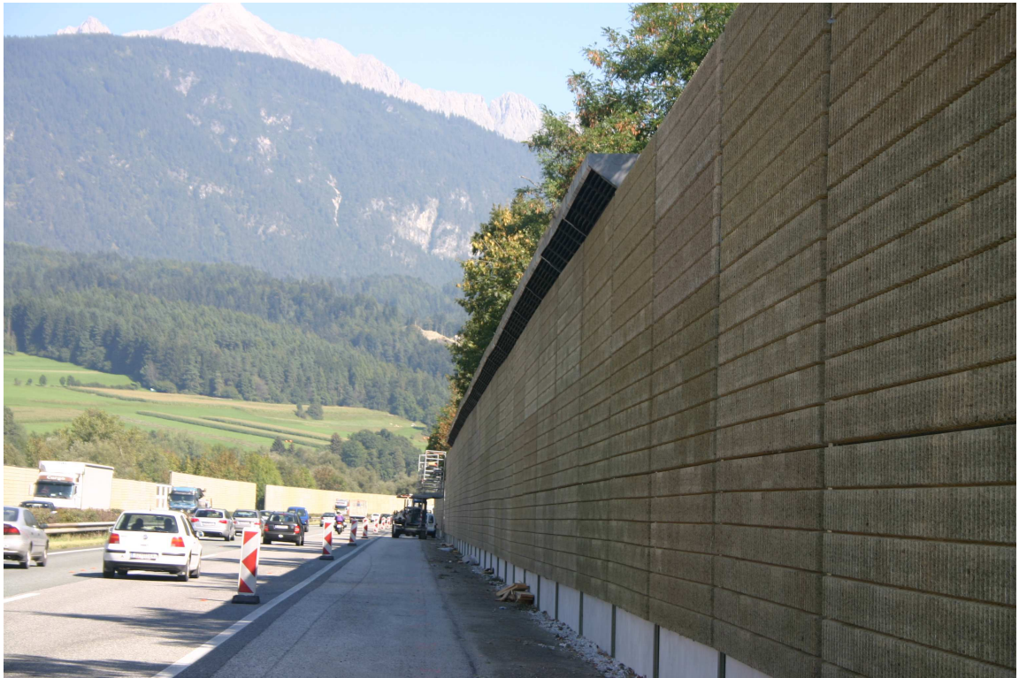
Fig. 1.6: Soundreducing headpiece (SSI: Sound Screen Improver) on a wall (near Innsbruck)
